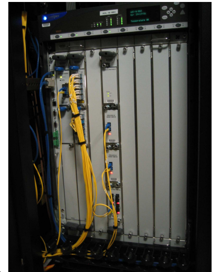
A Juniper router in use.
